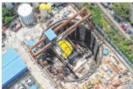
The heavy-duty machine is excavating from Sawli in Ghansoli towards Vikhroli and will dig a 10km stretch
